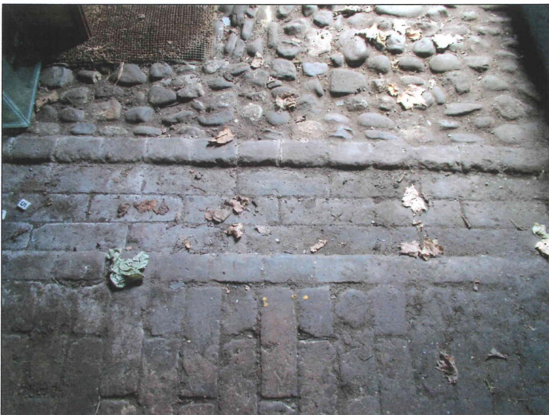
Plate 5 Drain and flooring in the coach room. Photo CPAT 1958-11
