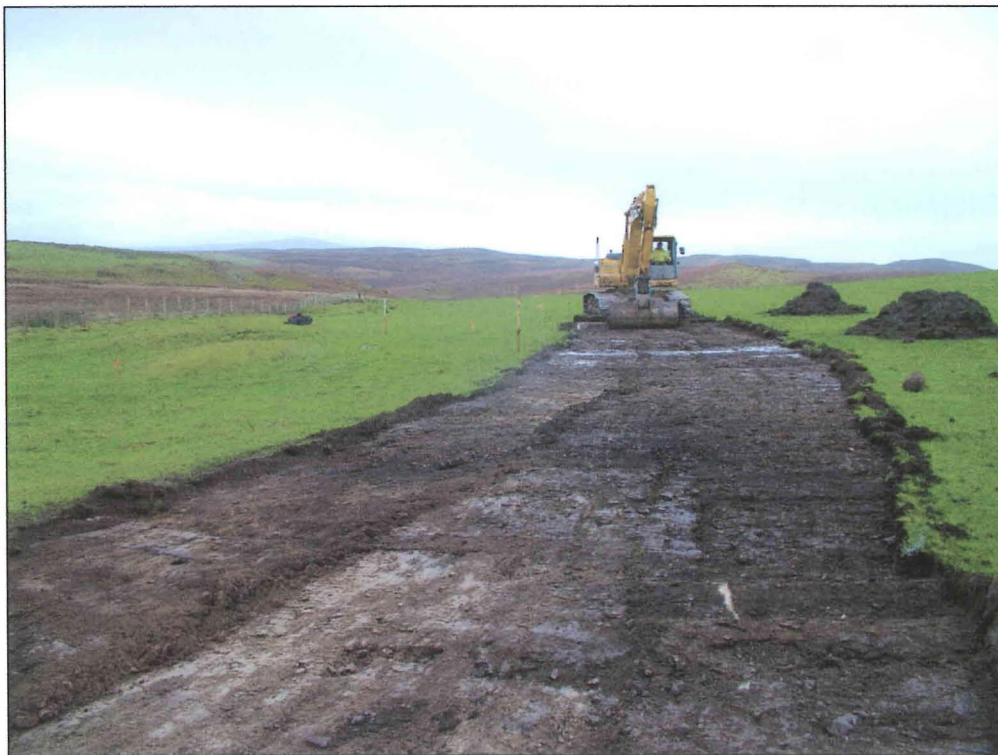
Plate 2 Topsoil stripping in the vicinity of the mounds (PRN 16971), (CPAT photo 2288-002)
