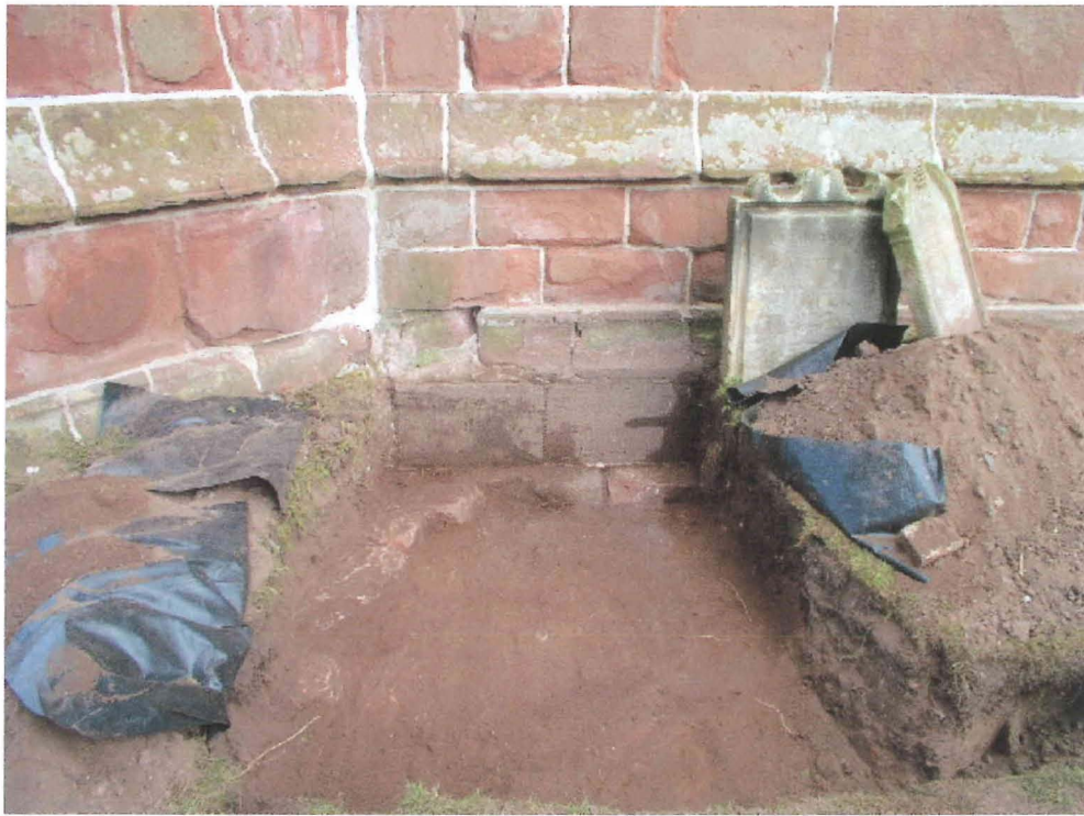
Plate 1 Excavated area against the west wall of the tower showing the stepped footings (4) and foundation (5) for the north-west buttress.
