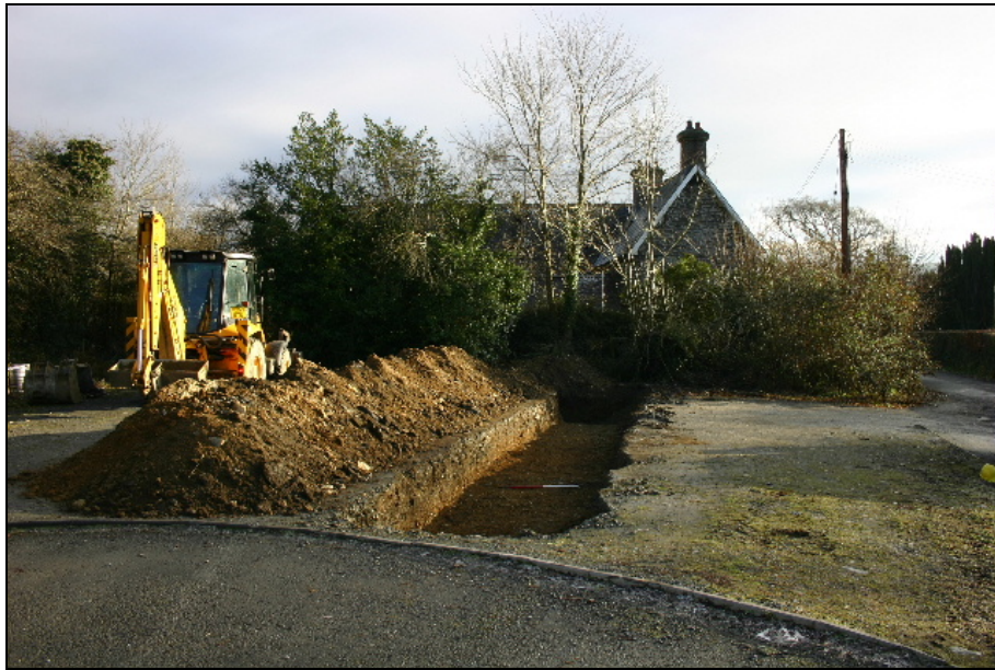
Fig. 4 Location of ground investigation works
