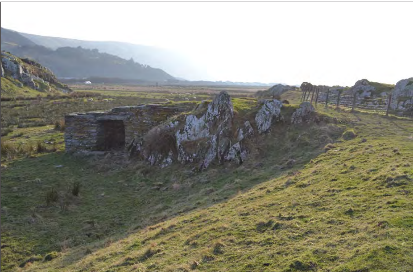
Plate 06: The Lime Kiln viewed from the east south east, showing hole into which the lime and fuel was shovelled. Scale 1m
