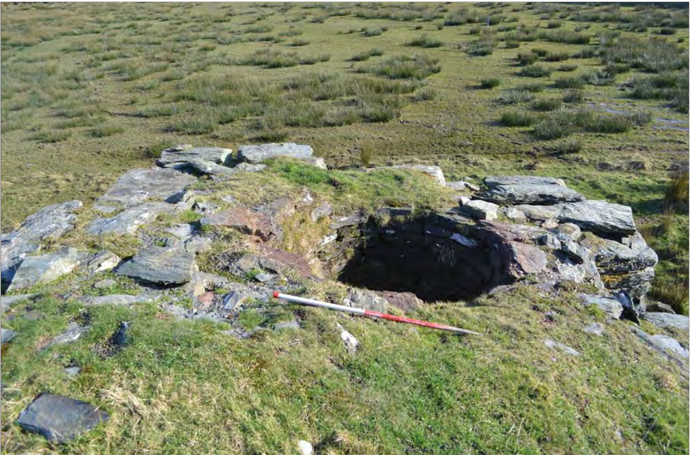
Plate 04: The Lime Kiln viewed from the north, showing hole into which the lime and fuel was shovelled. Scale 1m
