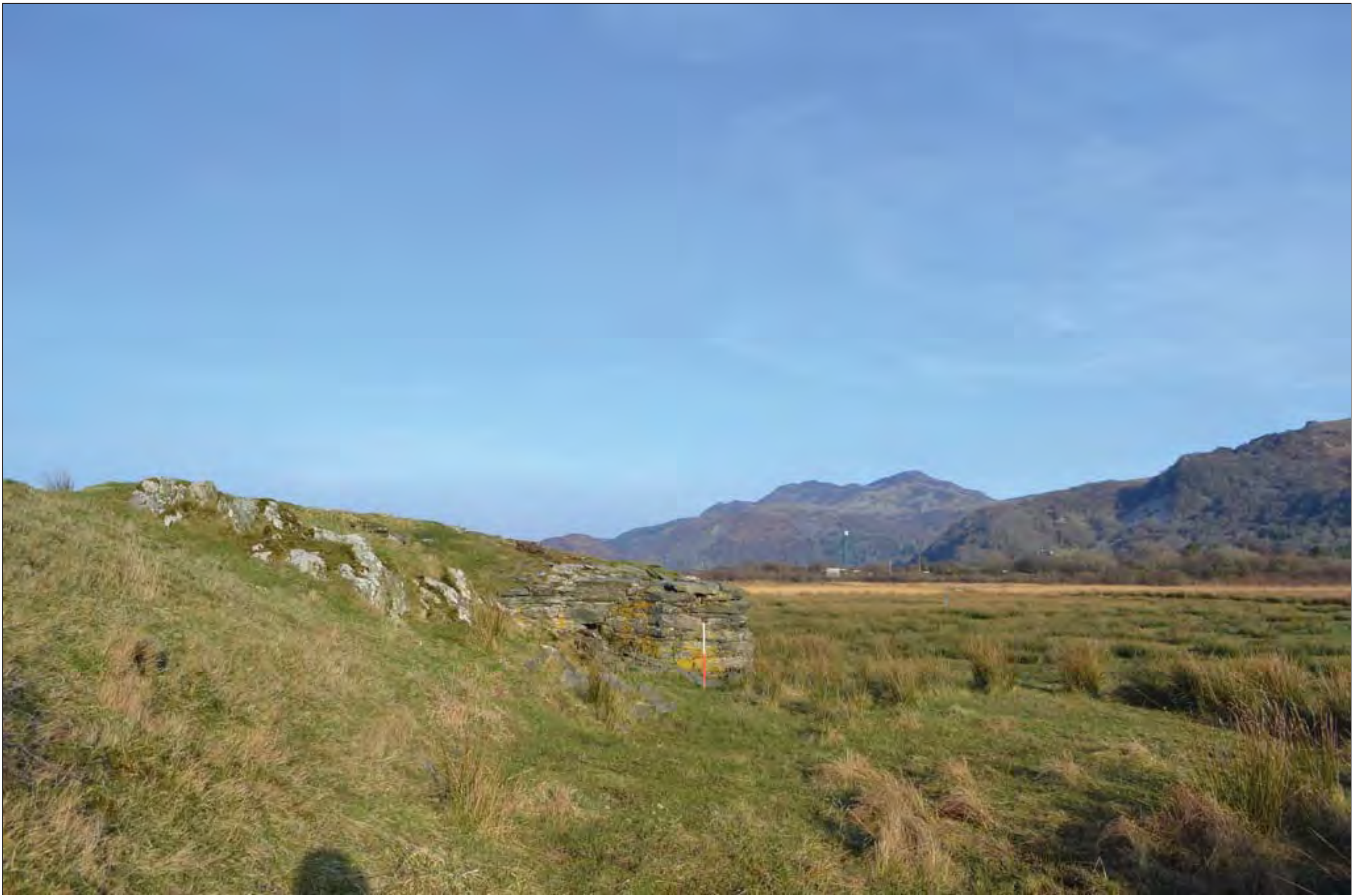
Plate 05: The Lime Kiln on the Fairbourne Embankment, viewed from the west, showing relationship with the rock outcrop built into the Fairbourne embankment. Scale 1m
