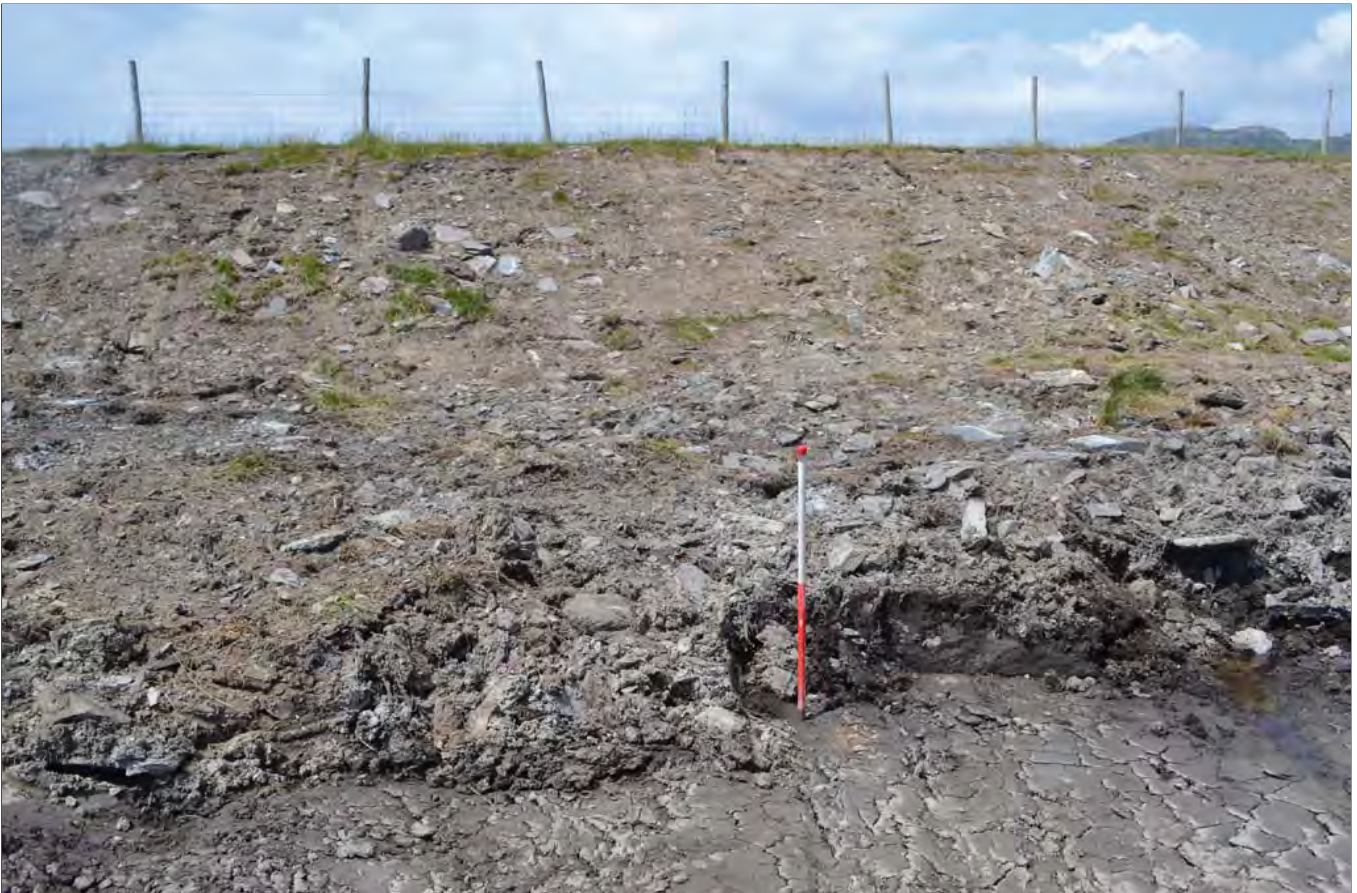
Plate 12: Fairbourne embankment, showing shale and clay make-up. View from the north. Scale 1m
