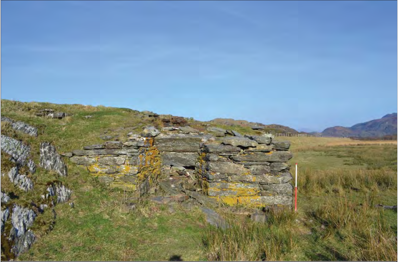
Plate 03: The Lime Kiln on the Fairbourne Embankment, viewed from the west. Scale 1m
