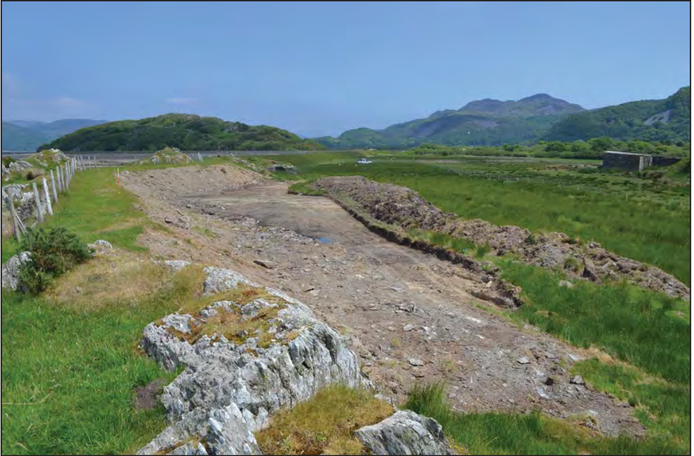
Plate 11: Topsoil strip adjacent to the embankment. View looking east
