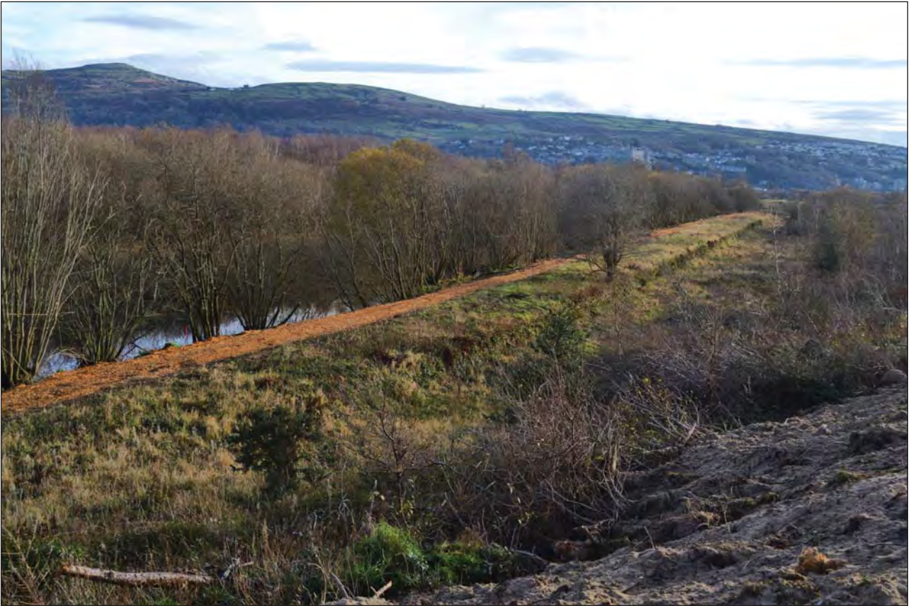
Plate 5. Southern end of the target railway embankment with Harlech Castle in the distance; view from NW (photo ref: G2790_082)
