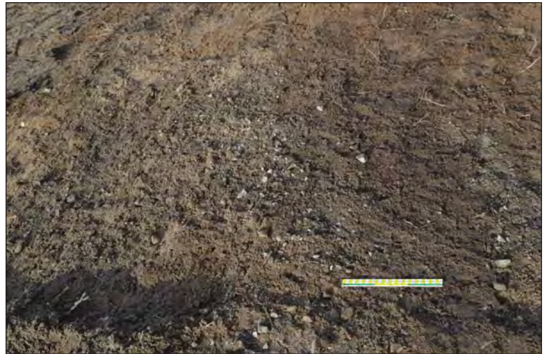
Plate 33. Cleaned up area of granite chippings forming railway track bed (context (06)); scale 0.3m; view from S (photo ref: G2790_068)
