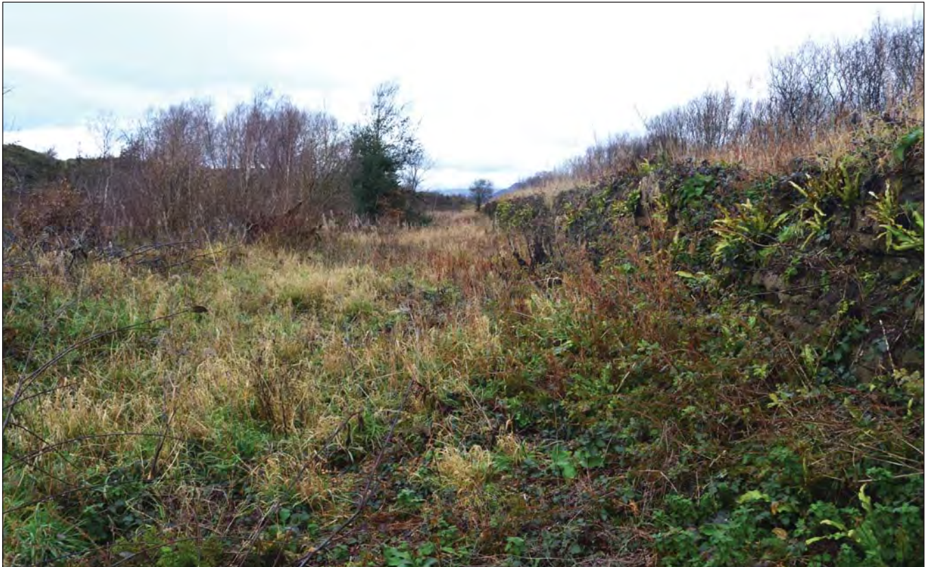
Plate 31. Location of railway running next to revetment of the southern part of the embankment; view from S (photo ref: G2790_011)
