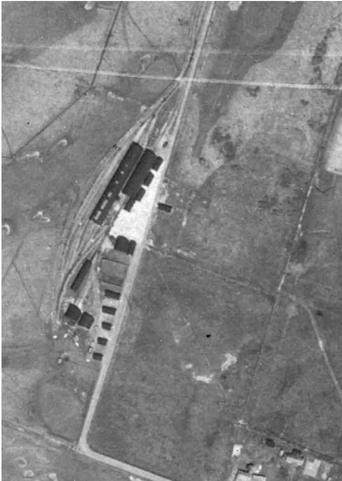
Engine sheds still in good condition and tracks still in place in 1946 (library no 4631, sortie RAF 106GUK 1468, frame 2414, date 04/05/1946)
