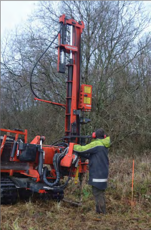
Plate 1. Hole being drilled for fence post (photo ref: G2790_100)
