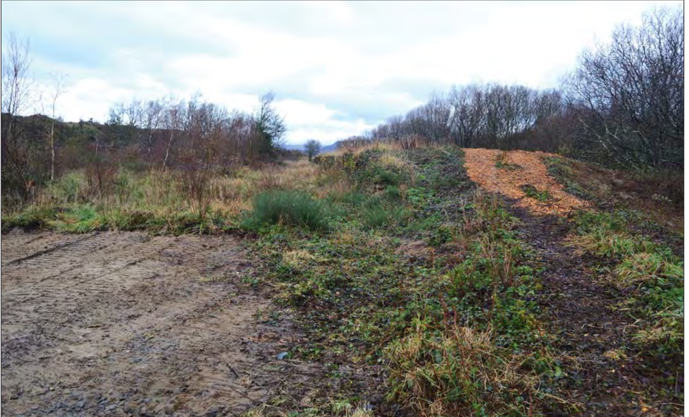
Plate 18. Ramp into southern end of embankment to allow access for forestry vehicles; view from SW (photo ref: G2790_008)
