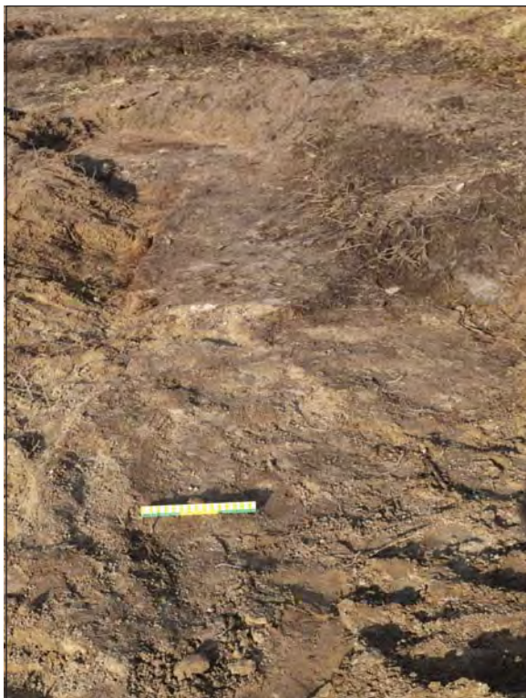
Plate 34. Concrete slab (03); scale 0.3m; view from S (photo ref: G2790_073)
