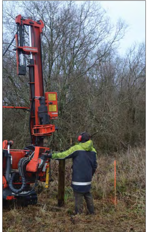
Plate 2. Fence post being driven into hole (photo ref: G2790_102)
