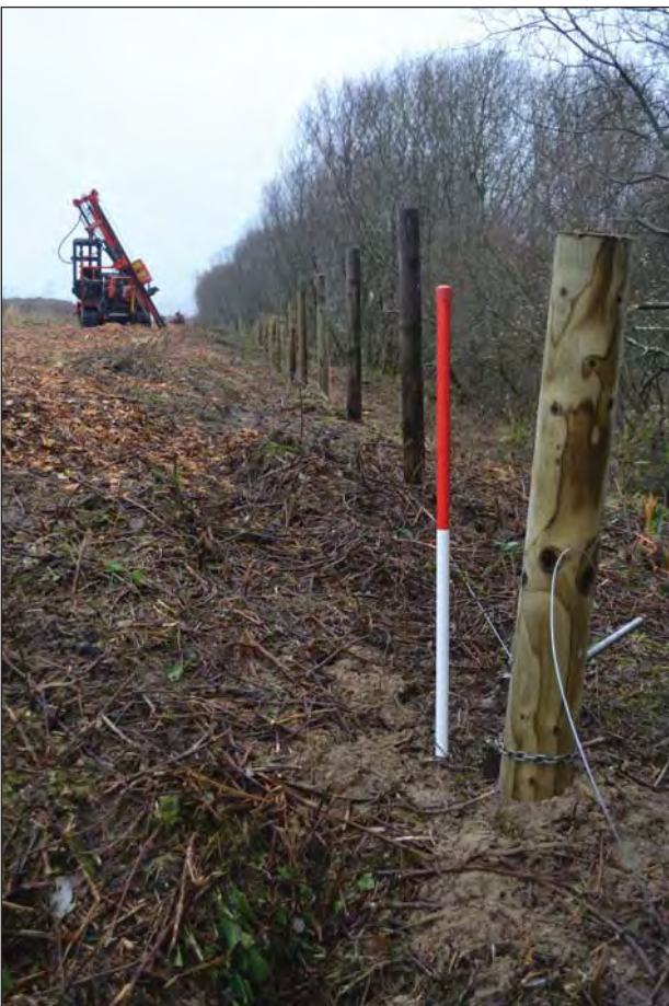
Plate 3. Example of fencing on embankment (photo ref: G2790_091)
