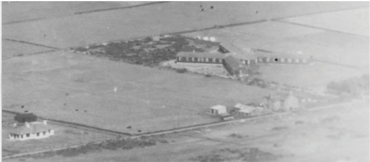
Oblique view of the buildings August 1941 (library no 4107/ M2962, sortie S/438, frame 110, date 24/08/1941)
