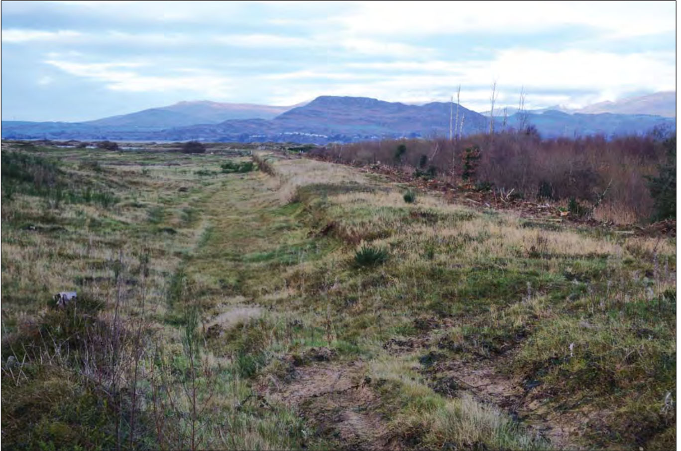
Plate 15. Target railway embankment north of sand encroachment with route of railway immediately to the left; view from S (photo ref: G2790_084)
