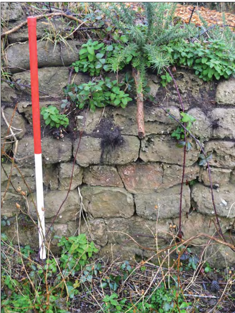
Plate 25. Heavily eroded and overgrown section of revetment; scale 1m; view from W (photo ref: G2790_012)
