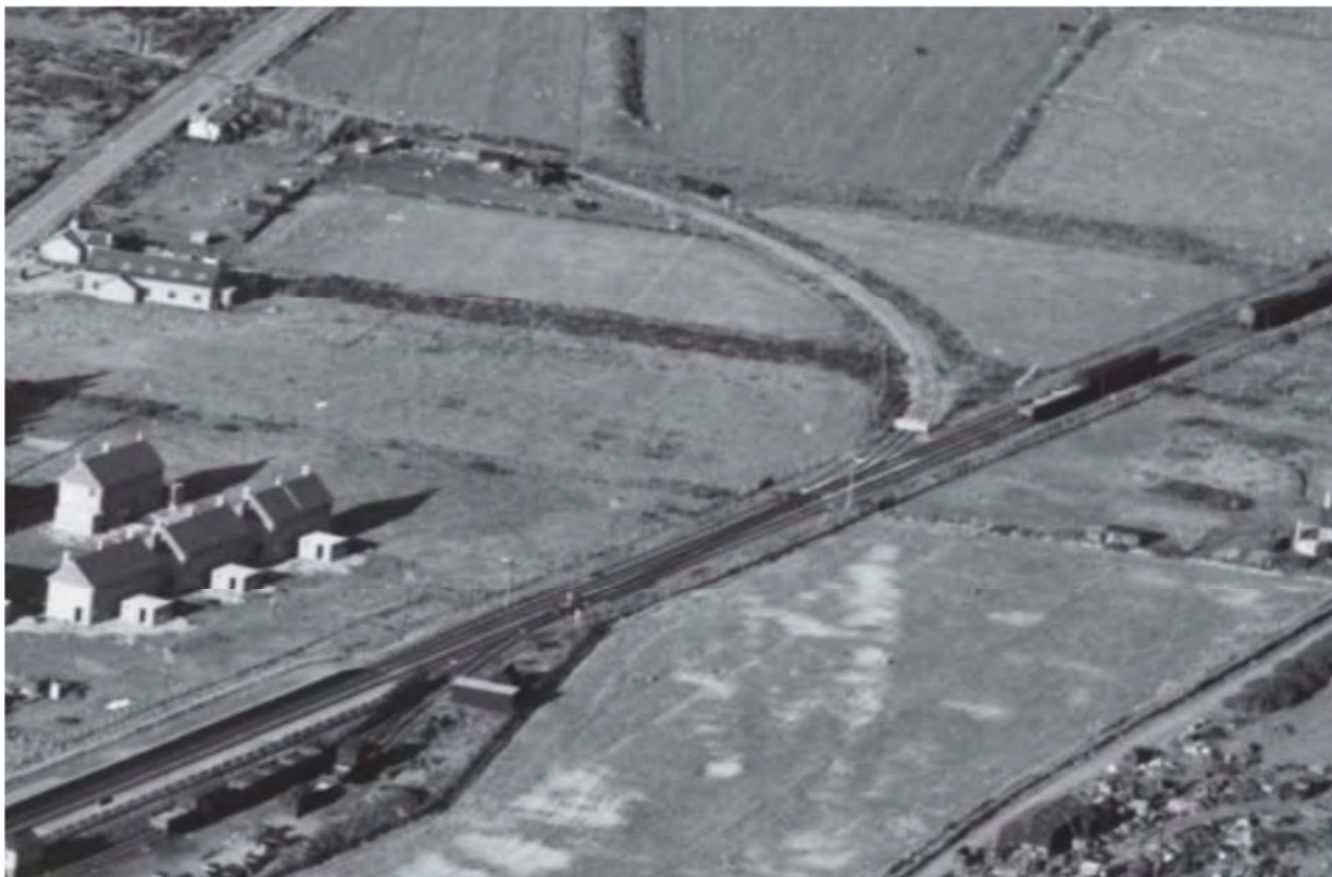
4. Rail siding leading to Military railway
