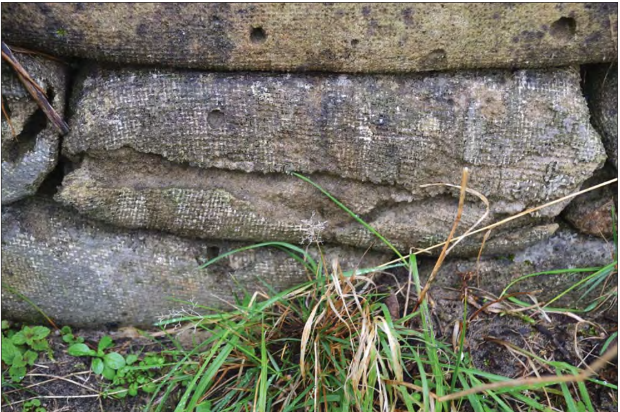
Plate 24. Cast of hessian sandbags in the concrete of the revetment; view from SW (photo ref: G2790_036)
