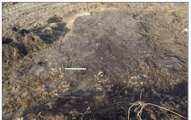
Plate 35. Concrete slab (05); scale 0.3m; view from S (photo ref: G2790_070)
