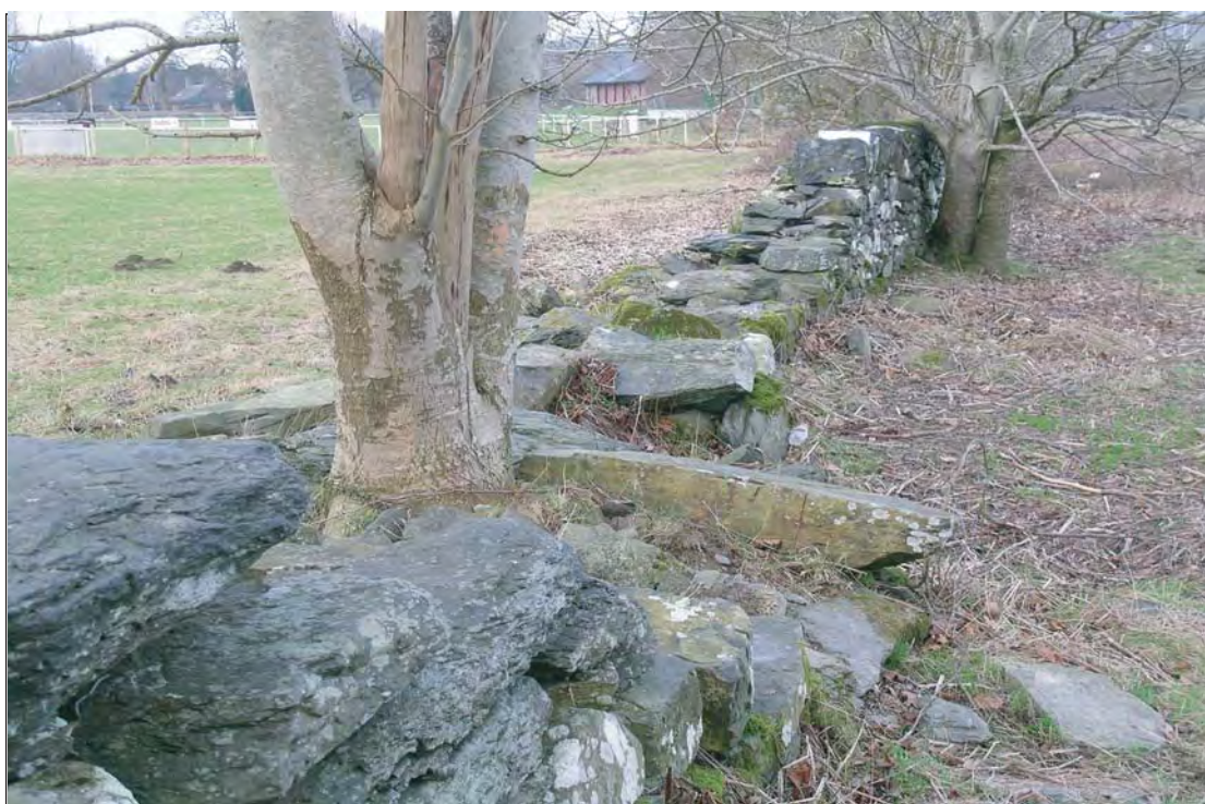
Plate 22: View North of Walkway/Boundary Wall
