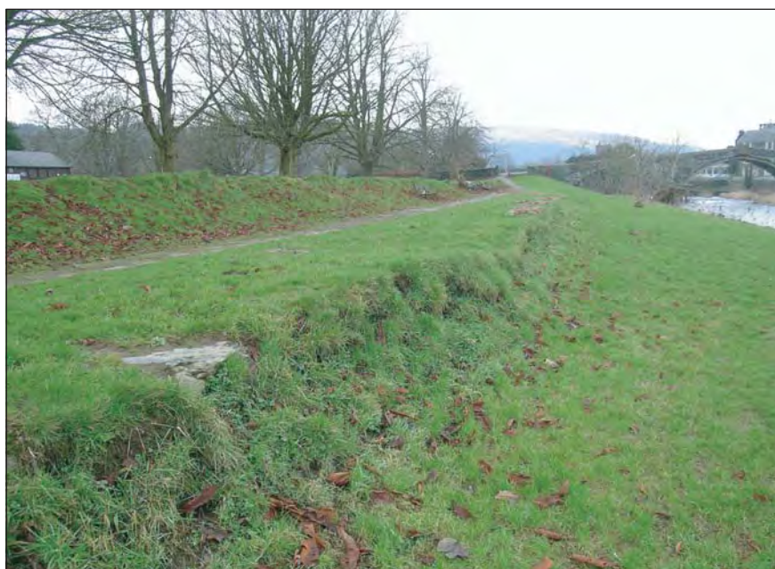
Plate 20: Terrace Line South of Bridge. Note Capping Stone of Wall Protruding From the Grass
