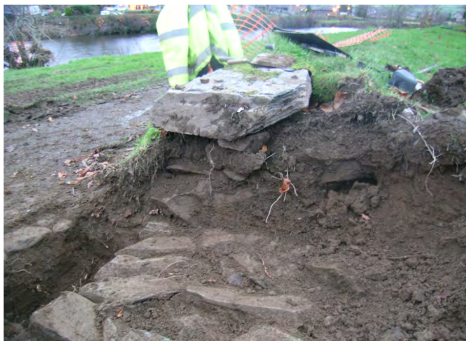
Plate 4: Section through Embankment Wall
