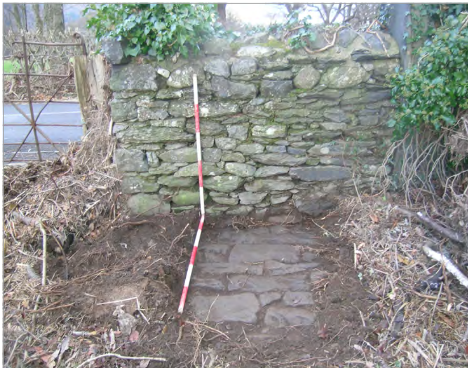
Plate 10: South facing Elevation of Trial Pit 1
