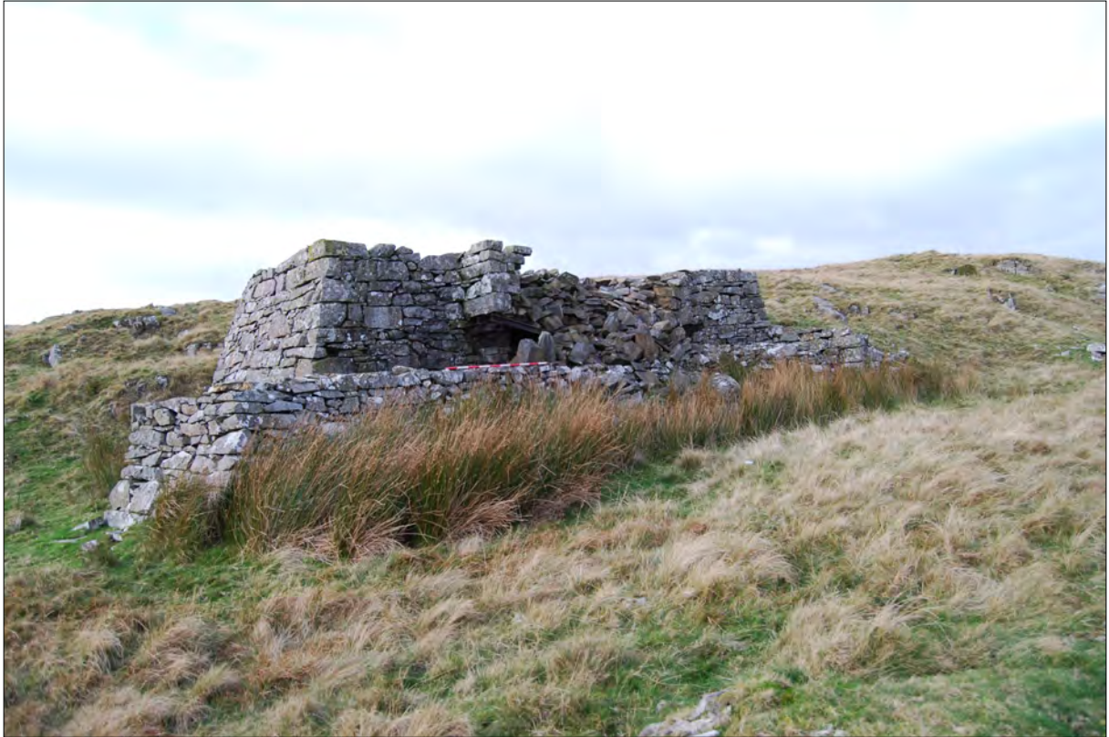
Plate 3. North west facing image of the Observation building showing the collapsed canopy.
