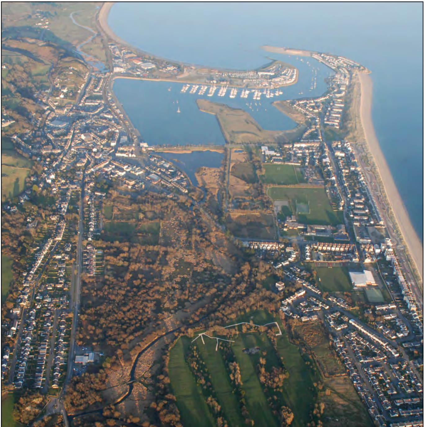
Aerial photograph of Pwllheli from the west which shows the original town built on a level terrace below Yr Allt
