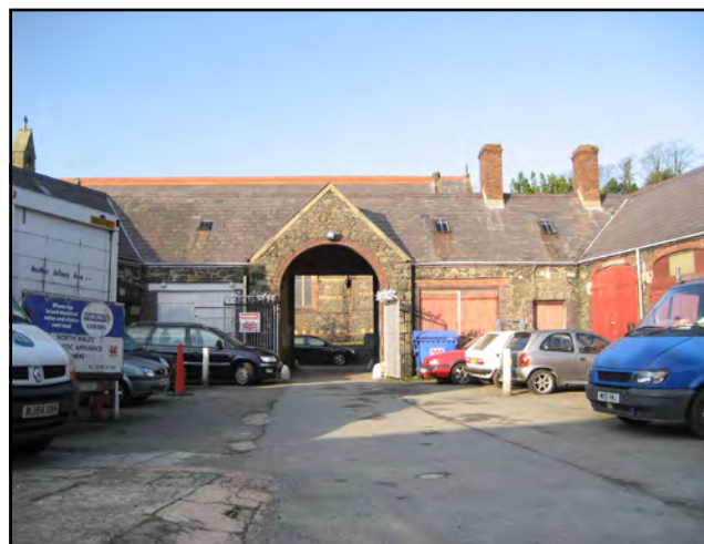
Coach stable yard behind The Tower
