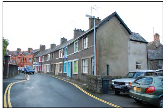
A row of pebble dashed buildings with door and window architraves on Ala street
