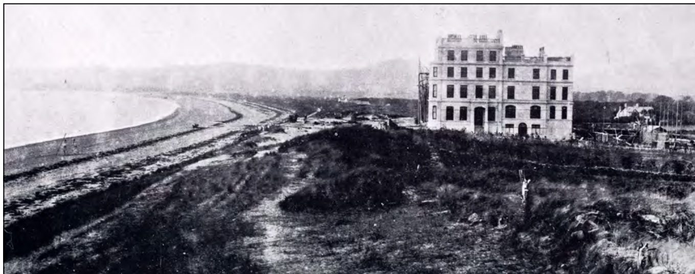
Soloman Andrews hotel at west end under construction 1898. (Andrews. J, 'The story of Soloman Andrews and his family, 1976, p.103)
