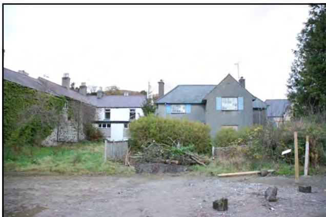
Semi derelict buildings behind Ala road
