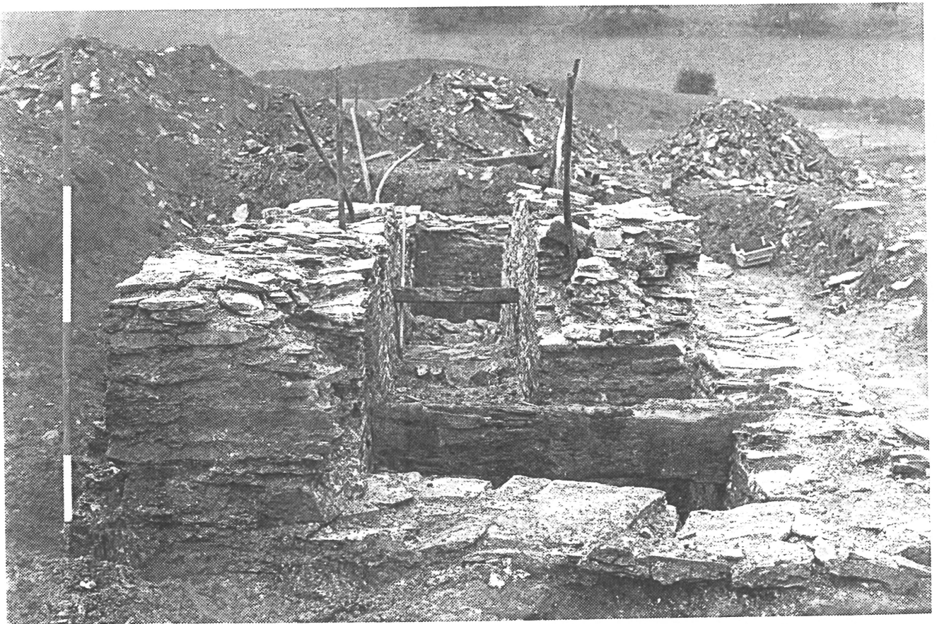
Plate 9: Building 29 from the northwest (2m scale)
