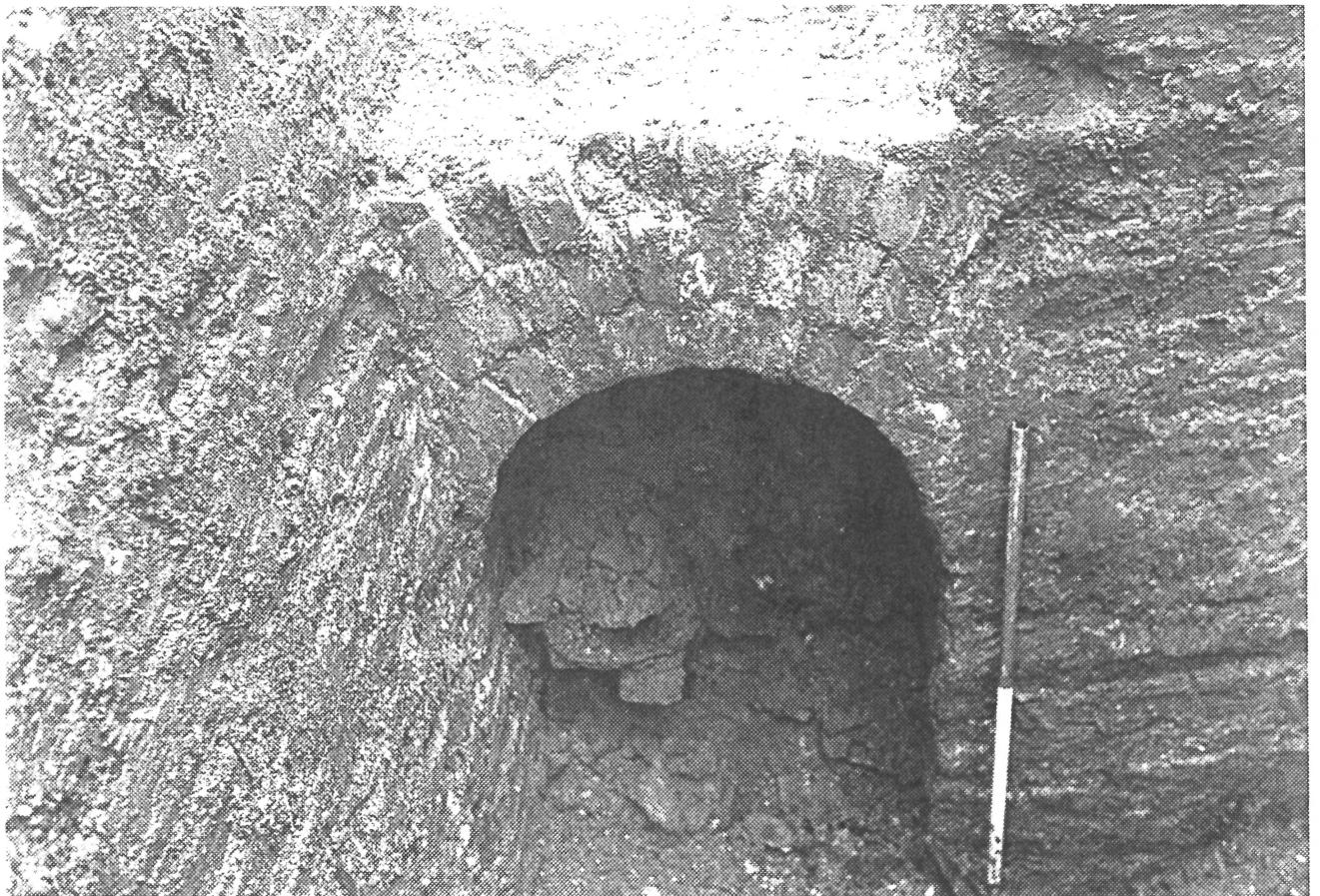
Plate 11: West end of the brick lined lower culvert (1m scale)
