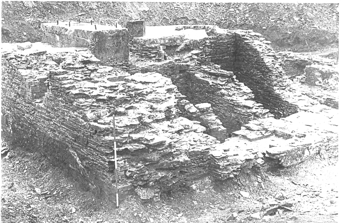
Plate 4: The number 30 engine house from the south (2m scale)
