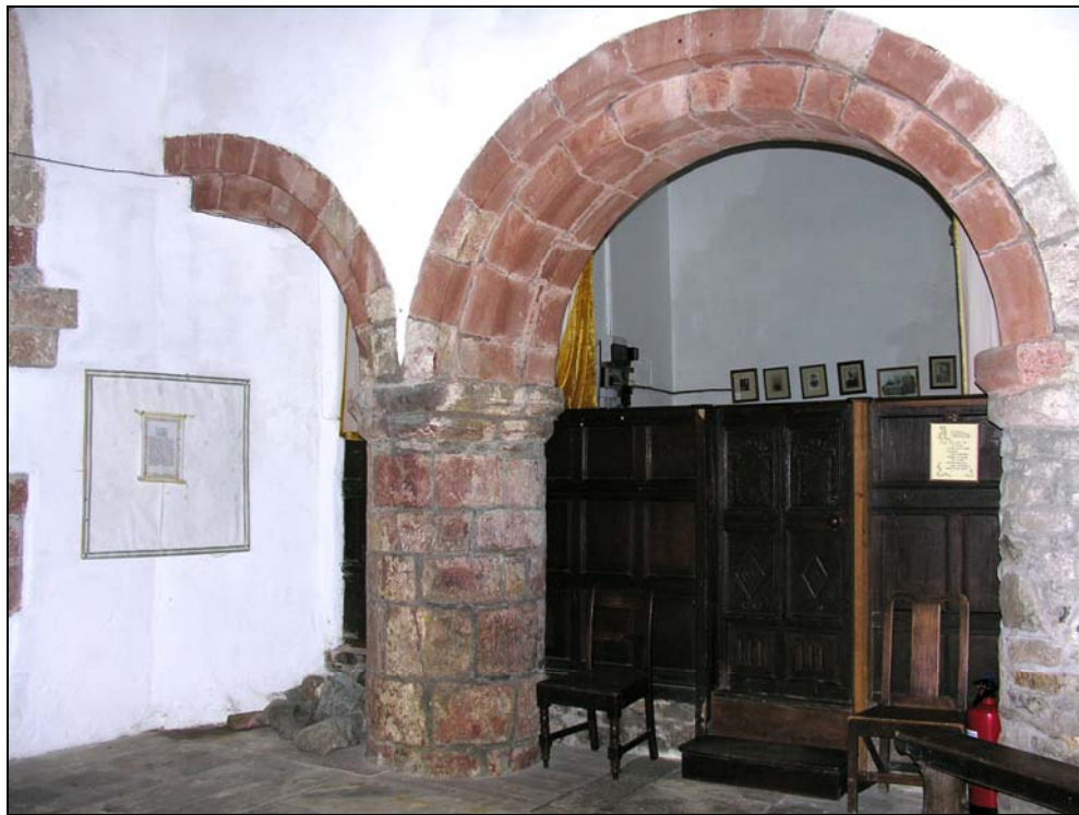
Fig 8: Shrewsbury sandstone used in Meifod church, Powys. © R J Silvester
