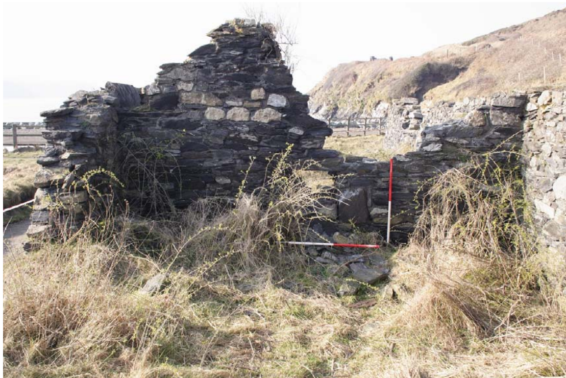
Plate 16: Cottage 3 west wall interior
