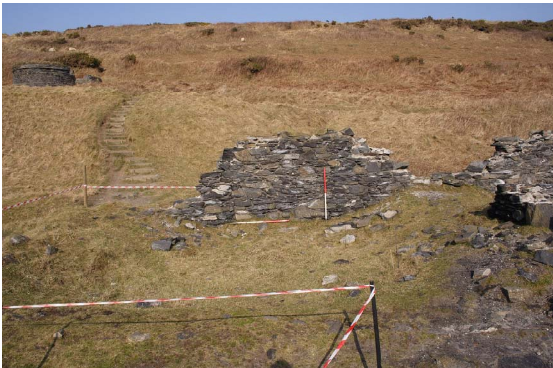
Plate 2: Cottage 1 north wall interior
