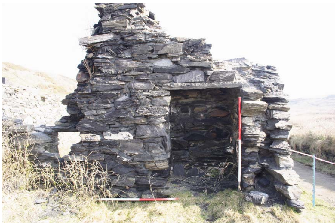
Plate 10: Cottage 2 east wall interior – detail of storage niche
