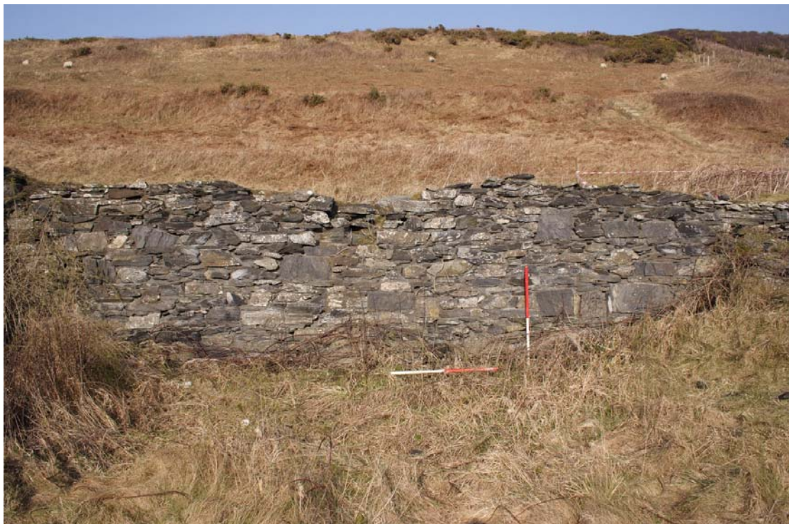
Plate 18: Cottage 4 north wall interior
