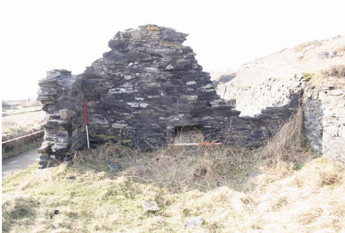
Plate 30: Cottage 6 west wall interior
