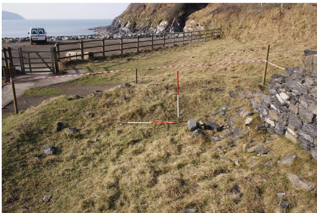
Plate 5: Cottage 1 west wall interior
