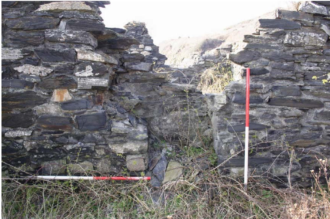
Plate 21: Cottage 4 west wall interior – detail of fireplace
