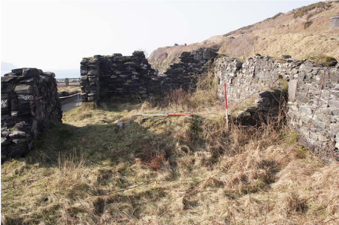
Plate 25: Cottage 5 west wall interior
