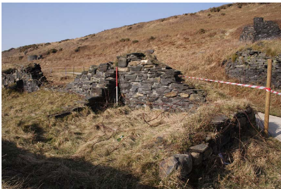
Plate 35: Cottage 7 extension north wall interior
