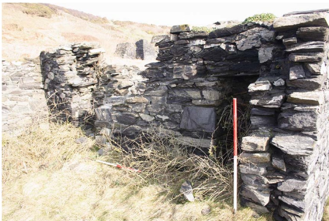
Plate 15: Cottage 3 east wall interior – detail of storage niche
