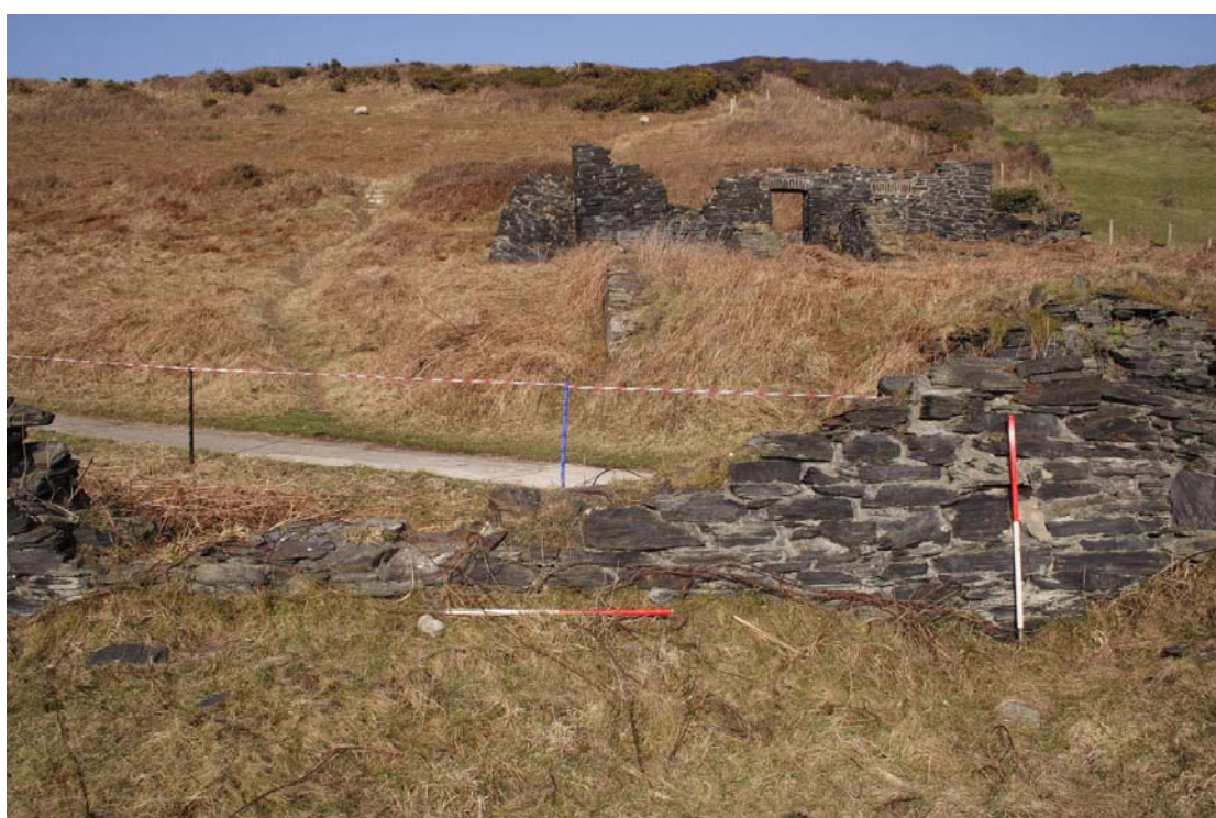
Plate 32: Cottage 7 north wall interior
