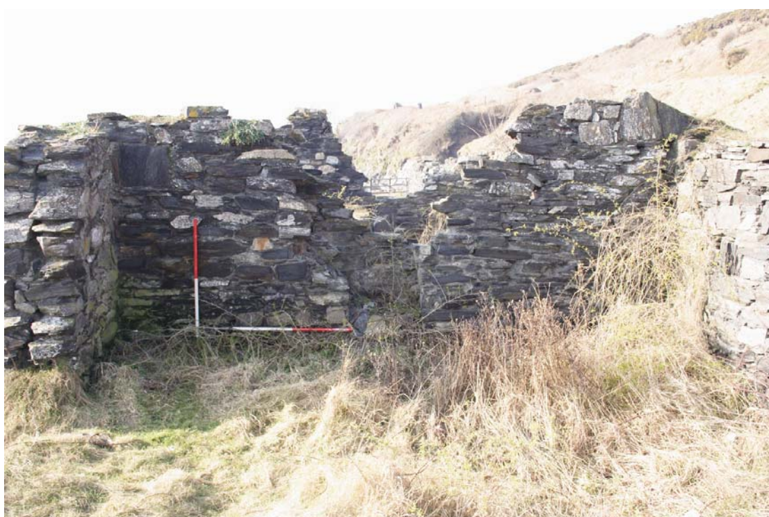
Plate 20: Cottage 4 west wall interior
