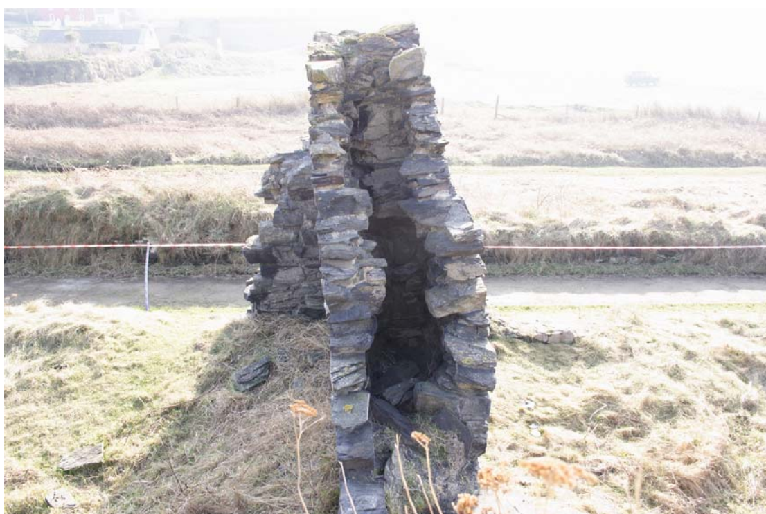
Plate 36: Detail of shared chimney between Cottages 5 and 6.
