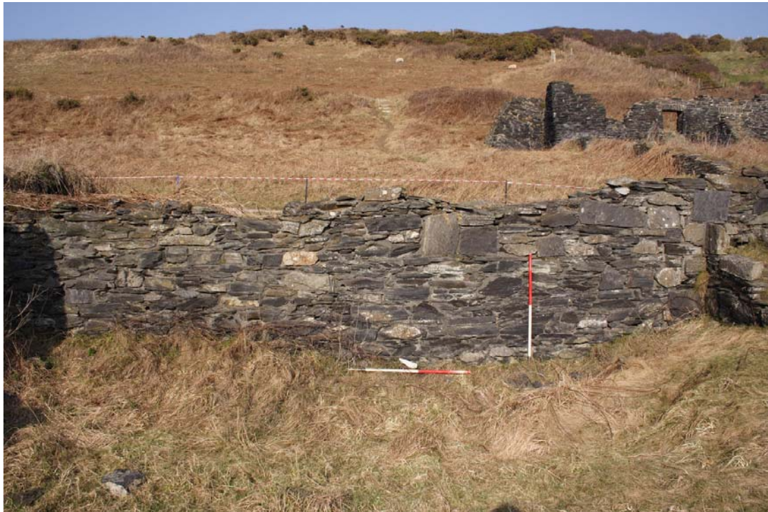
Plate 27: Cottage 6 north wall interior
