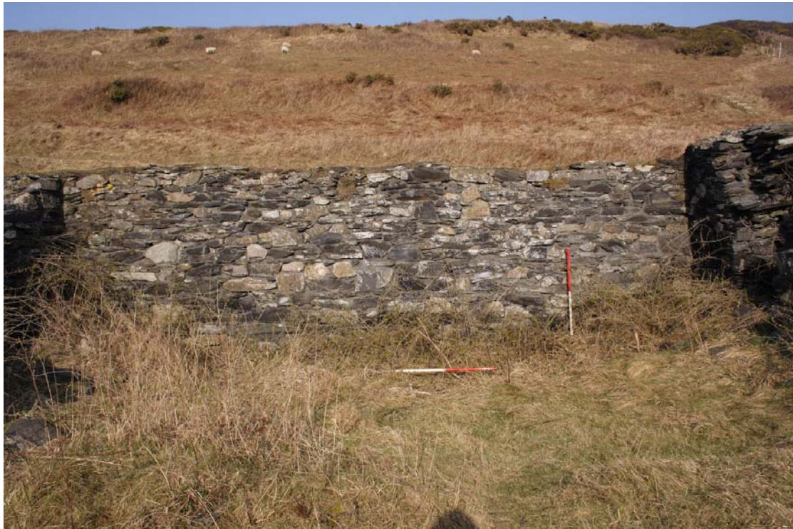
Plate 13: Cottage 3 north wall interior
