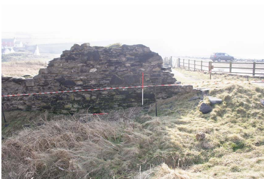
Plate 6: Cottage 1 north wall exterior
