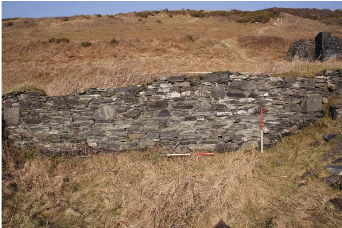
Plate 23: Cottage 5 north wall interior
