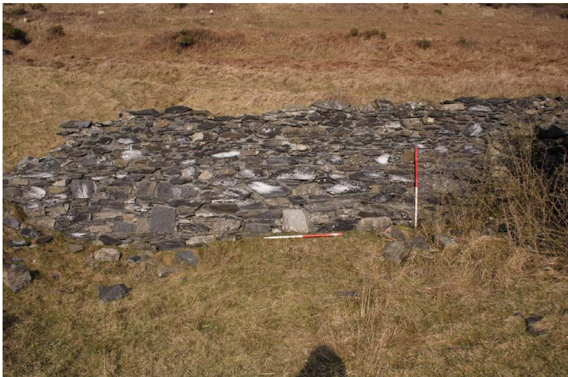
Plate 8: Cottage 2 north wall interior
