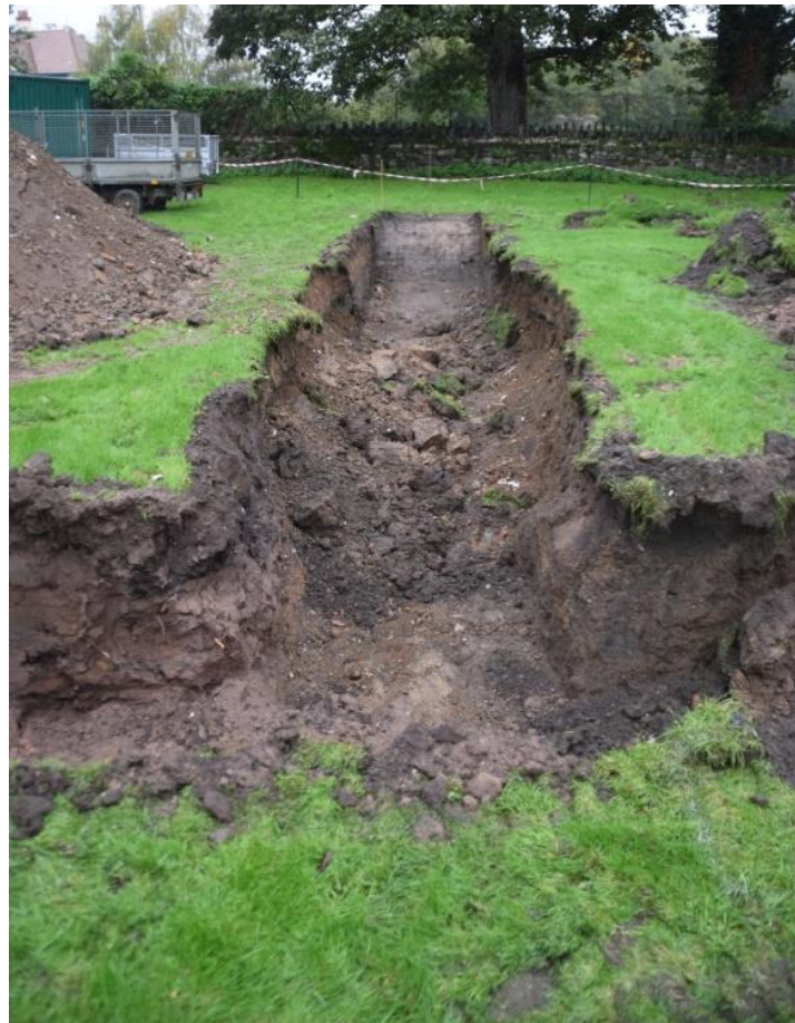
Figure 14: Trench 3 collapse
