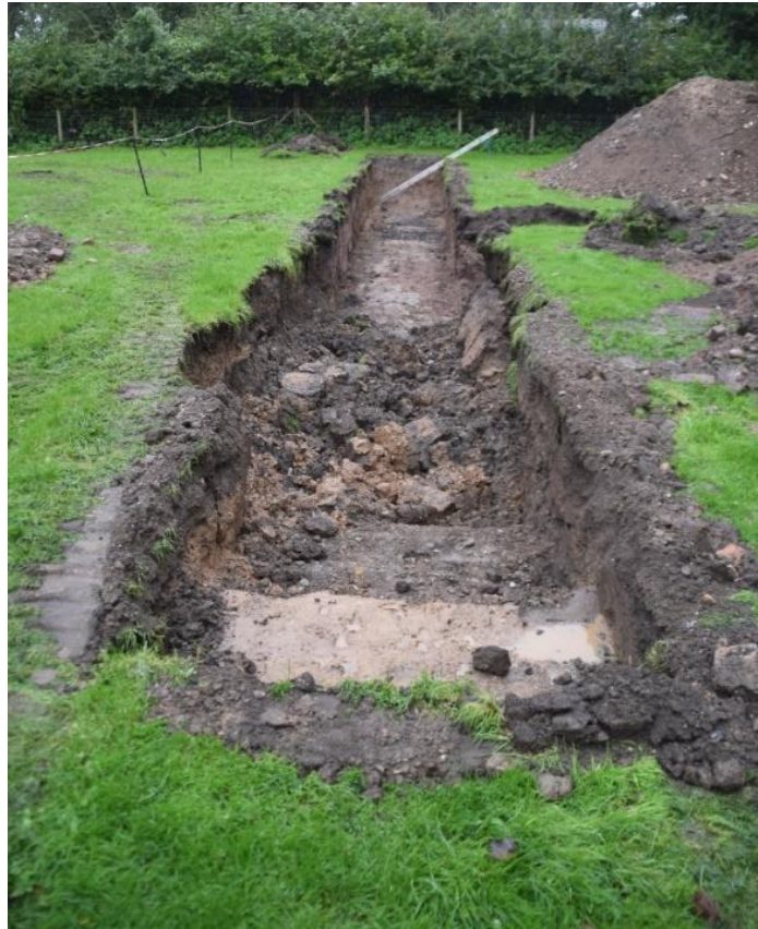
Figure 15: Trench 4 collapse
